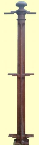
This piece of the Planter was part of the bridge balustrade replaced during restoration
